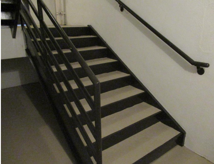
6. Handrails in Stairwell Overview
