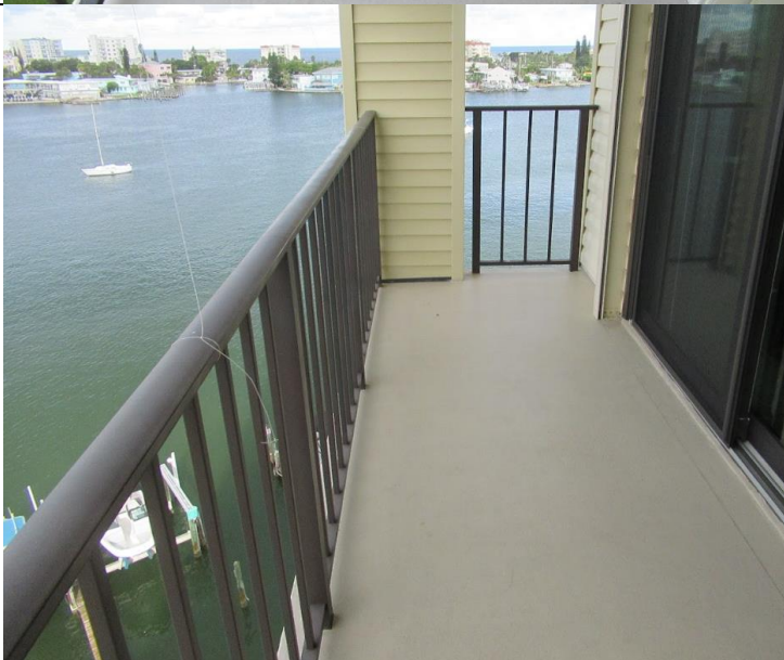
8. Unit Balcony Overview
