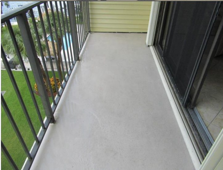
7. Unit Balcony Overview
