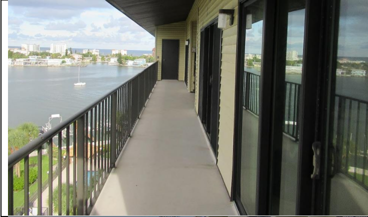
9. Guard Rail Balcony Overview
